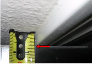
Use a flat straight surface, and place against thickest portion of door trim. Measure thickness of trim nearest the wall from edge of surface to the wall, keeping all angles square and mark distance as shown.
