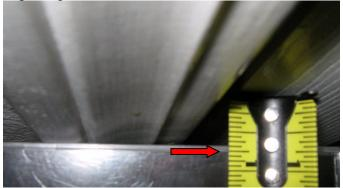
Measure thickness of trim nearest the door from edge of surface and mark as shown. The difference between these two measurements is the difference in the plane, and should not be greater than 9/16 inch.
